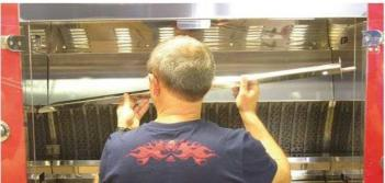
•First presents the end of the spindle in the bearing located on the left of the double wall unit
